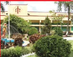
UNIT NO. 1 NASIK PLANT
