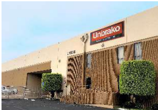
West Coast Distribution Center
