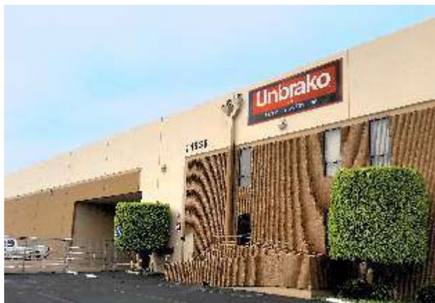
West Coast Distribution Center
